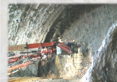
Lattice girder and shotcrete are used in the construction of the underpass
